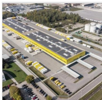
ENNS/LINZ CROSS DOCK
